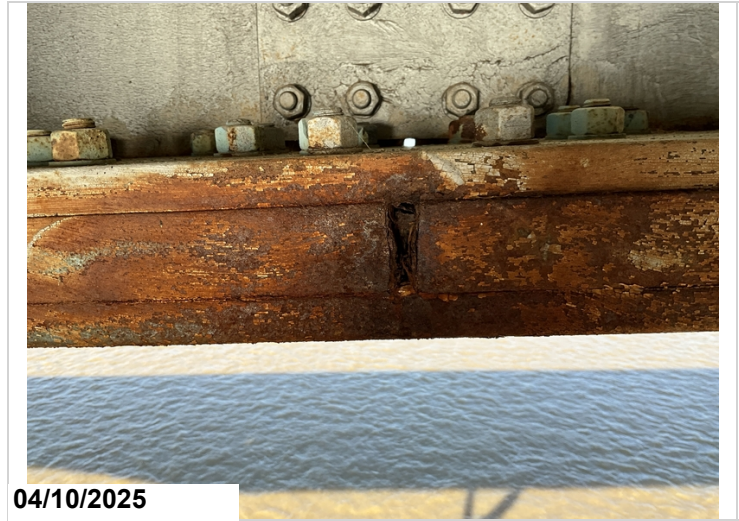
Span 56, girder 1, 1st splice plate connection, right side: active corrosion, 1/16" section loss, 1LF CS2.
