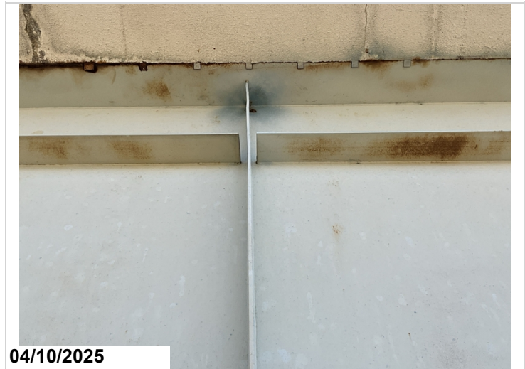
Span 57, girder 1, left, floorbeam 15, vertical stiffener: out of plane bending, 1LF CS2..
