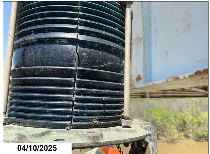
Span 57, left blue navigation light has broken fixture which allows moisture inside .
