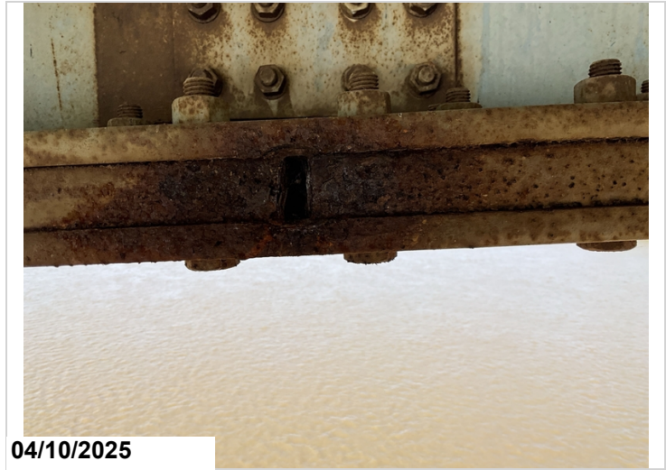
Span 56, girder 1, right side, 2nd splice plate connection: active corrosion with section loss, 1LF CS3. Up to 1/16" section loss, this typical at girder 2.
