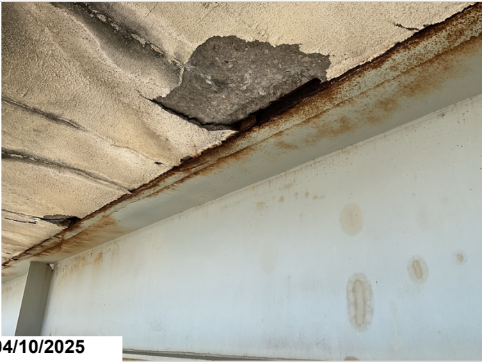
Span 56, girder 2, right side, top flange, between floorbeams 6 and 7: active corrosion with section loss up to 1/8" 7LF CS3.
