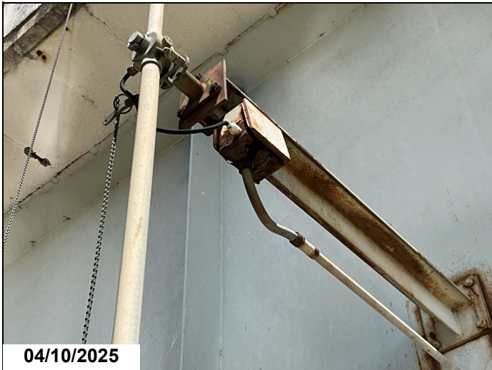
Span 57, left side, 3rd nav light: electrical junction box is completely rusted through, typical at all other nav lights
