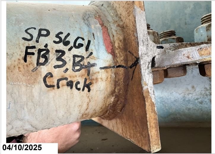
Span 56, floorbeam 3, girder 1, bottom, back side, diagonal connection plate: crack on both sides of plate, cracks are 1/4", CS3.
