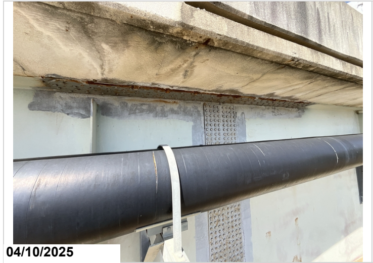
Span 56, girder 2, right side, 3rd splice plate connection: active corrosion, 10LF CS2.
