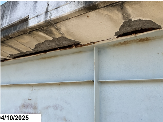
Span 56, girder 1, left side, floorbeam 6, top flange: corrosion with section loss 15LF CS3. Up to 1/8 section loss.
