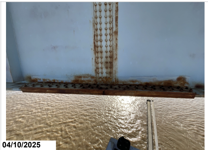
Span 56, girder 1, 1st splice plate connection, left side: active corrosion, 10LF CS2.
