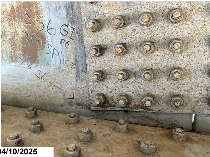
Span 56, girder 1, left side, 3rd splice connection: up to 3/16" old section loss, 1LF CS3. 2"x10" area.
