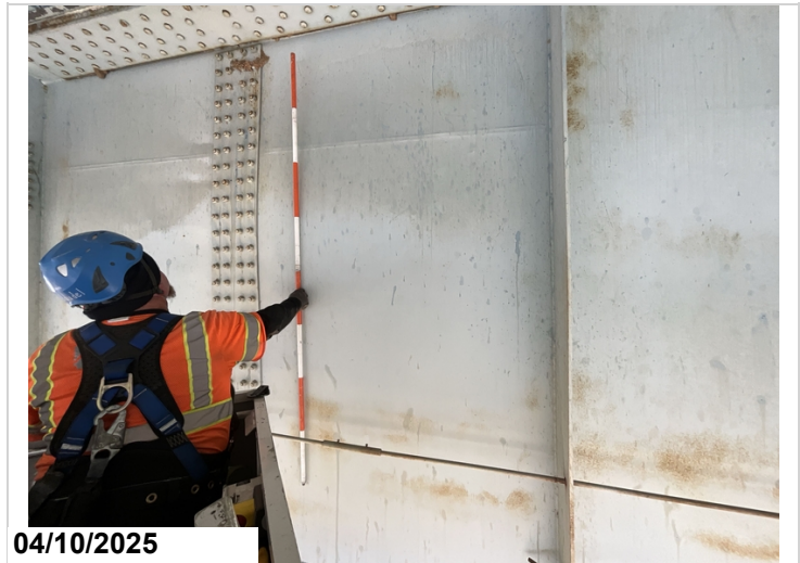
Span 56, girder 2, 1st splice connection: out of plane bending, 13LF CS3
