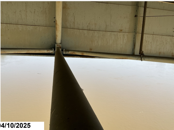
Span 57, floorbeam 20, bottom transverse member: out of plane bending, 10LF CS2.
