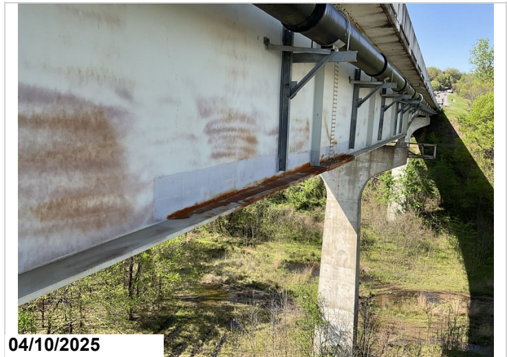
Span 58, girder 2, right side, at 3rd splice connection: surface corrosion, 20LF CS2
