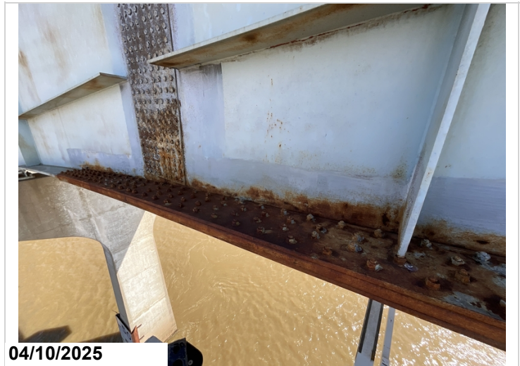
Span 56, girder 1, left side, 3rd splice plate connection: active corrosion, 10LF CS3.
