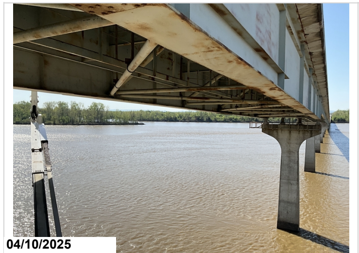
Span 56, typical condition of protective coating.
